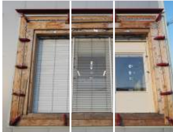
Shading system control
